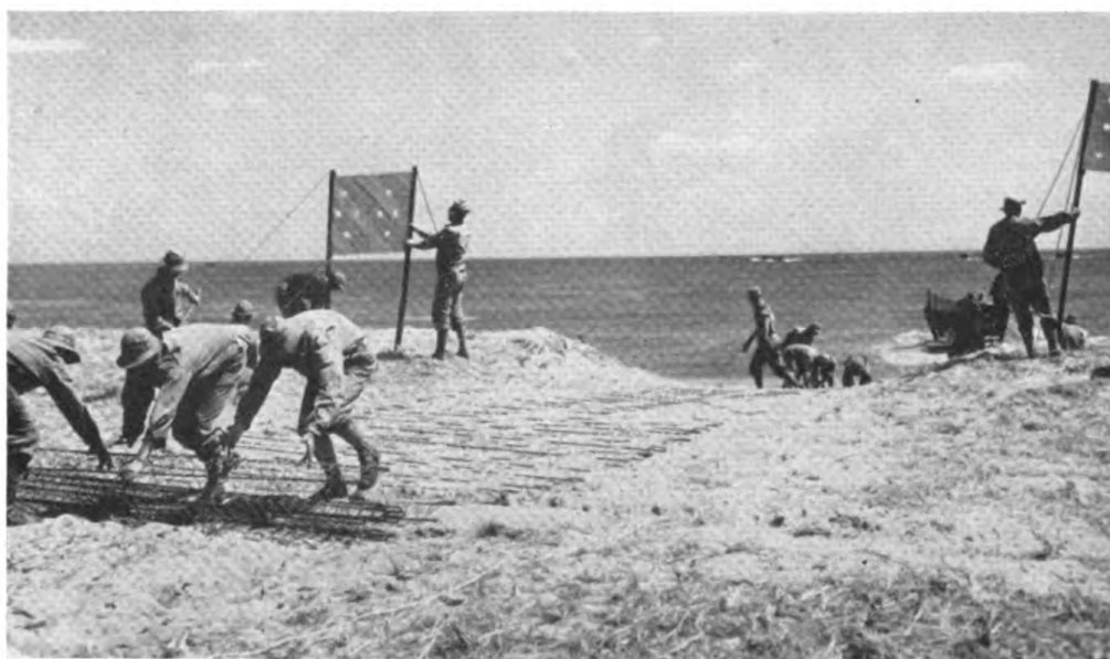
Shore engineers install markers and prepare a roadway at Cape Cod in 1942. (Signal Corps photo)
