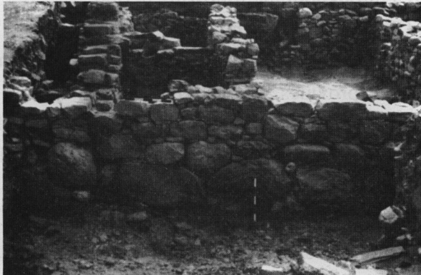
Fig. 13: Terrace wall with foundations contruted form limestone and basalt boulders.
